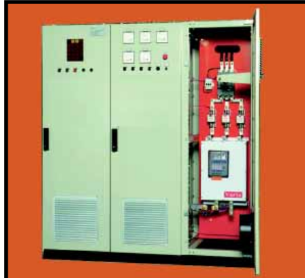
STATIC EXCITER WITH VEC 205E, FOR 5000 KVA SYNCHRONOUS GENERATOR
